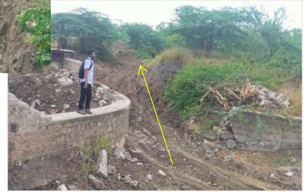
Excess soil taken out
